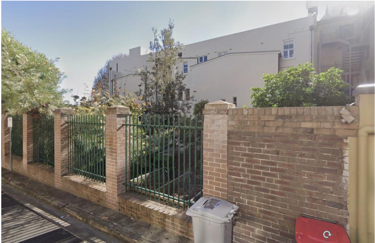
Figure 13: Rear of Garcia building as viewed from Rockwall Lane facing northwest
