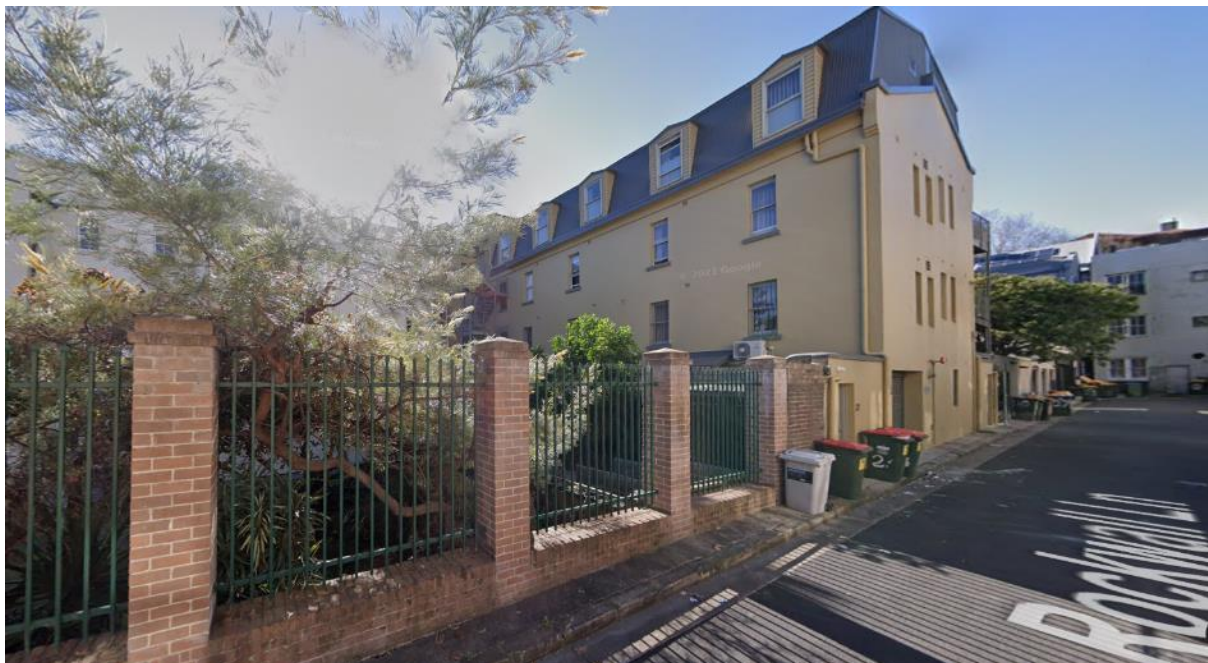
Figure 12: View looking northeast to the rear of Hotel Challis and Garcia building from Rockwall Lane
