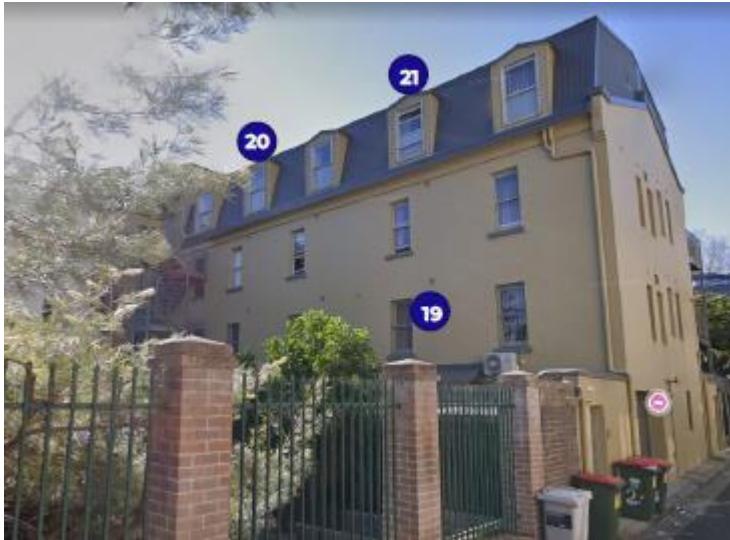
Figure 76: Extract from VLA identifying three hotel rooms selected for view loss assessment and corresponding CAM No.
