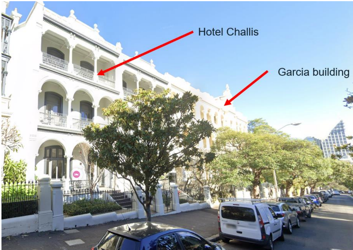
Figure 11: View looking southwest along Challis Avenue
